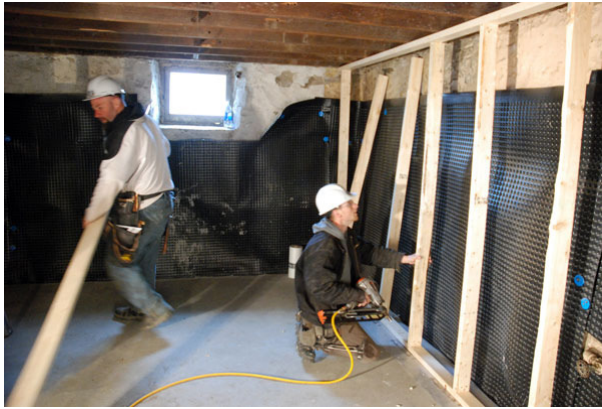
Insulating the basement
